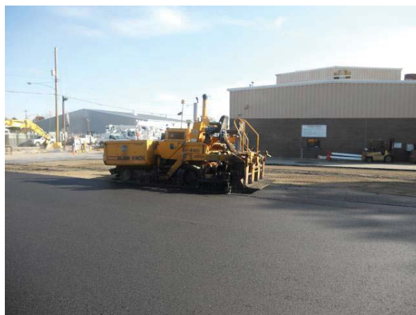
Paver used to place base-course
