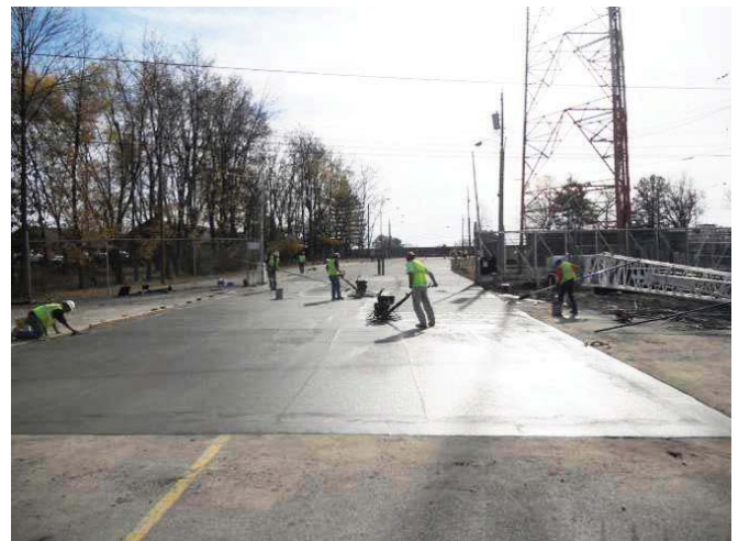
Finishing work on new concrete pavement
