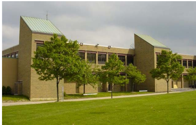
Overview of Harrison High School project in progress.
