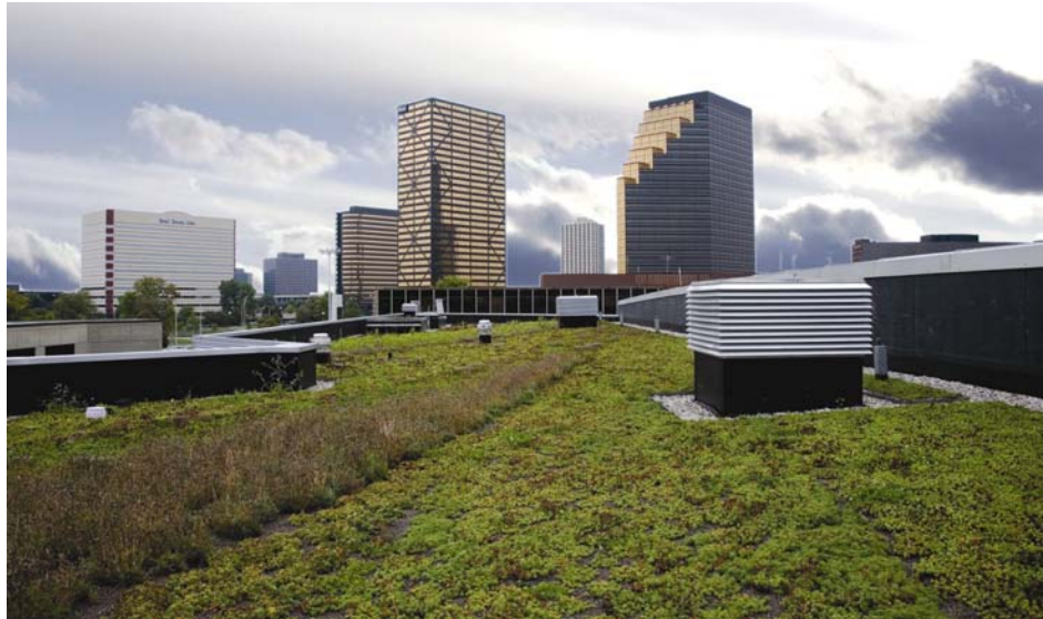
Overview of green roof
