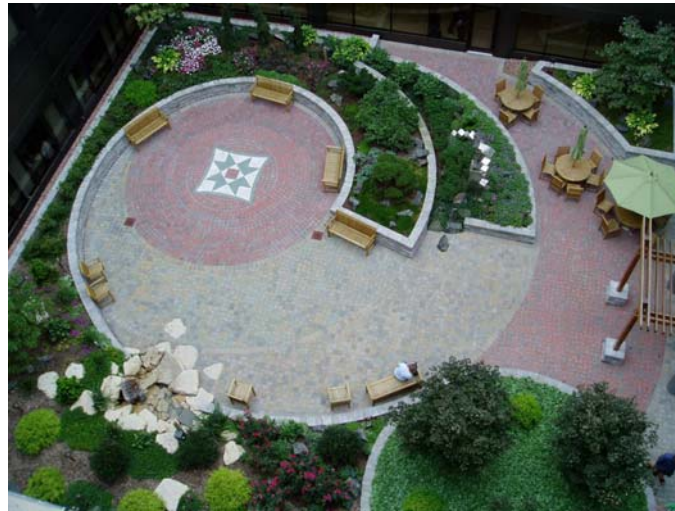
Plaza Waterproofing / Green Technology
