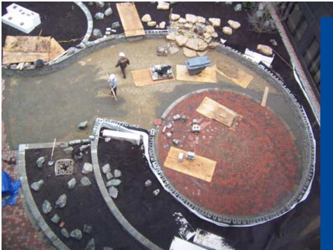
Installation of duel layer system during construction phase
