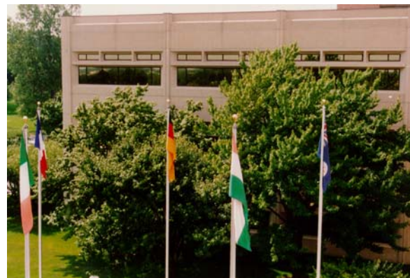
Overview of World Headquarters Precast Concrete Panels
