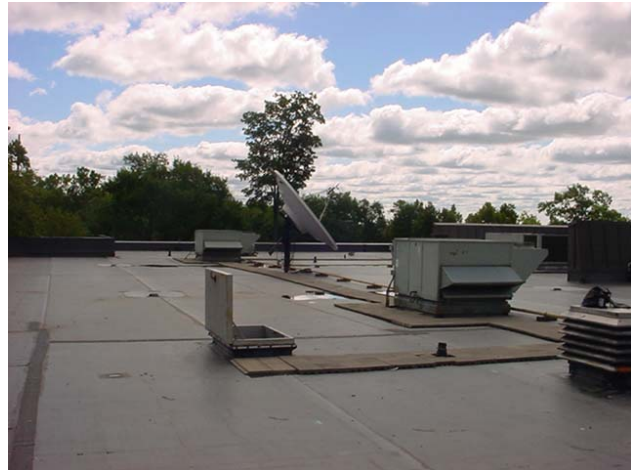
Overview of completed roof replacement.
