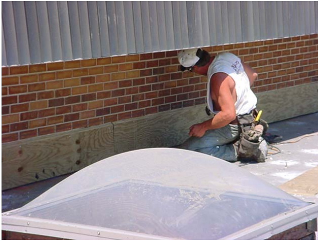
New baseboards with proper flashing were installed along the parapet wall.
