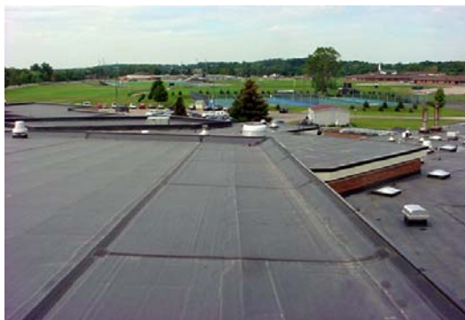
Overview of roof replacement
