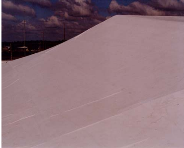
Close-up of CSPE hypalon on Portage Central Middle School
