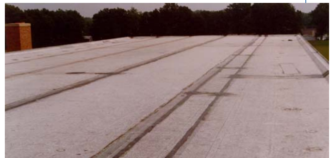
Overview of completed field of roof - Low Bay
