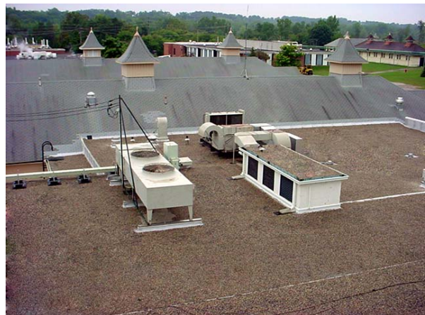
Overview of completed roof replacement
