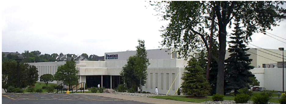
Overview of Parkedale Pharmaceutical Complex
