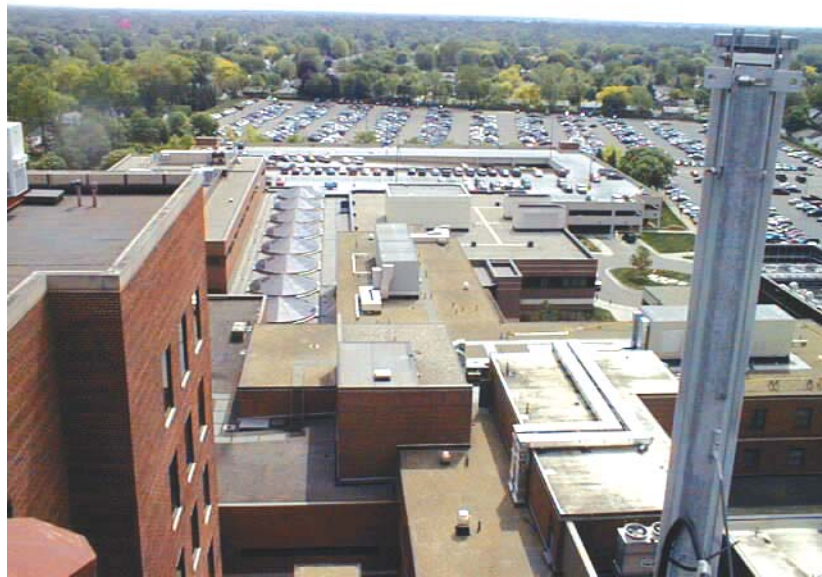
Overview of various roof areas at Oakwood Hospital & Medical Center.
