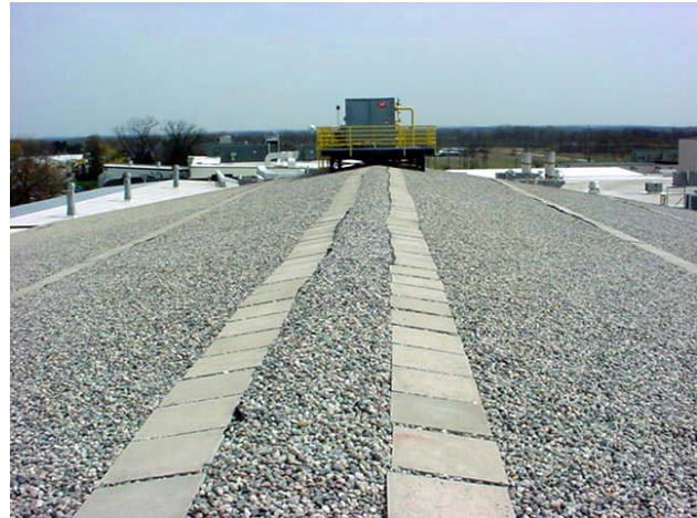
Overview of completed reconstruction.
