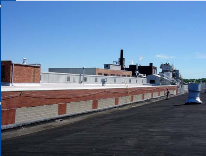
Overview of facility prior to work commencing.
