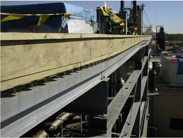
New structure was constructed over and around existing building.
