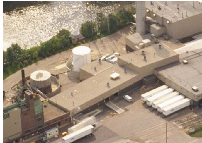
Overview of the completed new building.
