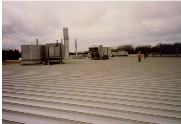
Overview of field of roof
