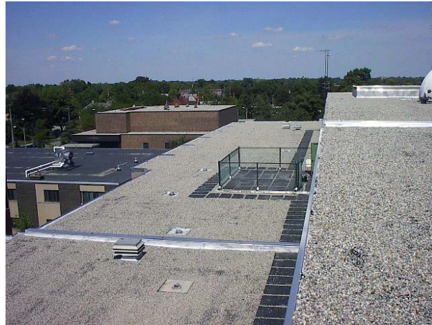
Overview of completed roof replacement project.
