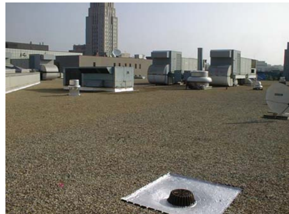
Overview of completed roof replacement.
