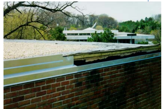
New fascia system was designed with careful attention to detail to allow for perimeter movement.
