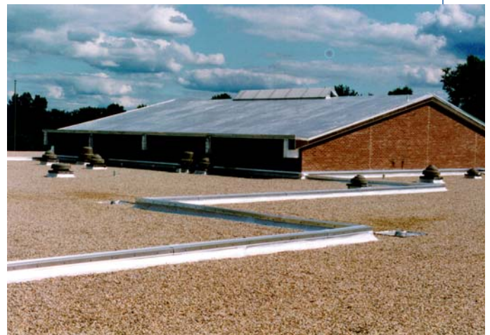
Completed installation of built-up roof system
