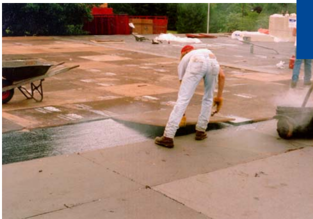
Installation of second layer of insulation.
