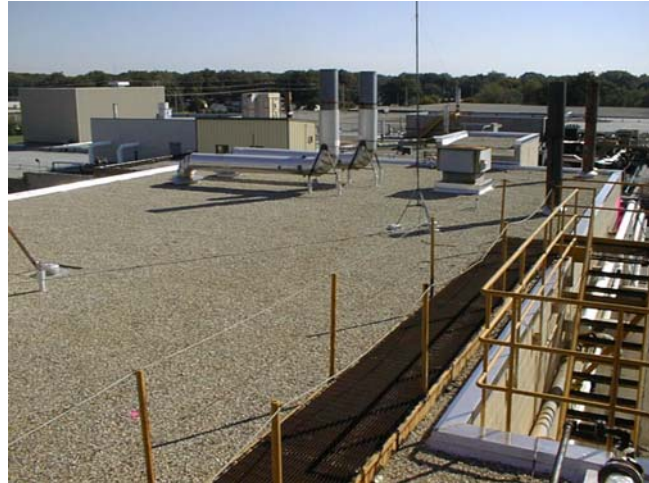
Overview of completed roof replacement.
