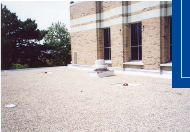
New drains and sheet metal flashings demonstrate attention to detail.
