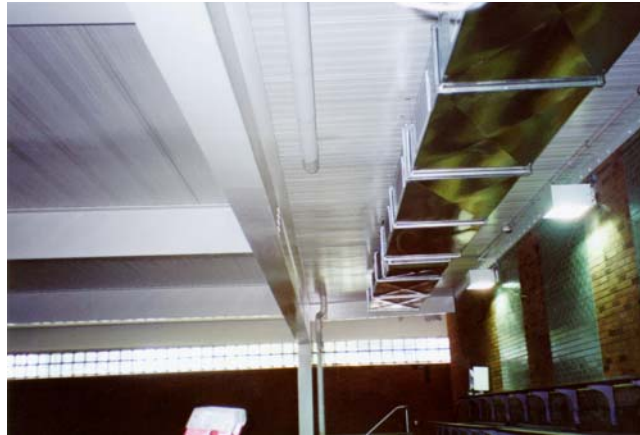
New steel deck and restored structural steel beams were cleaned and painted.
