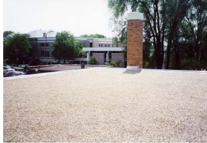
Overview of completed roofing project.
