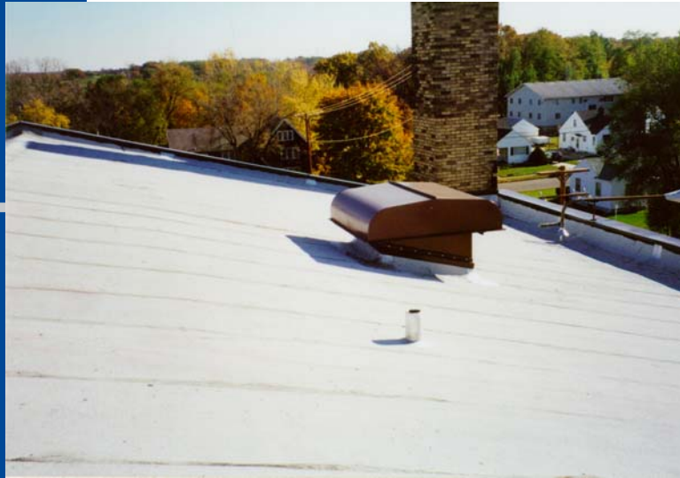
Overview of completed roof replacement.
