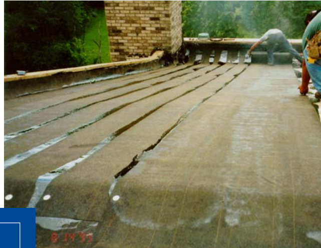
Bituminous plies were installed overlapping and fully adhered.
