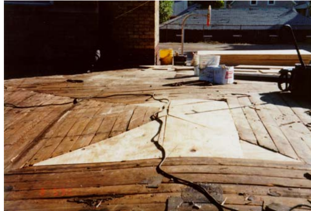
Deteriorated wood decking was replaced with new lumber.
