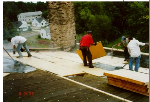
Fully-adhered insulation board is being installed.
