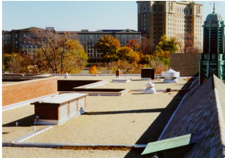
Overview of completed low slope and steep slope roofing.
