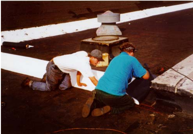
Work in progress on the expansion joint.
