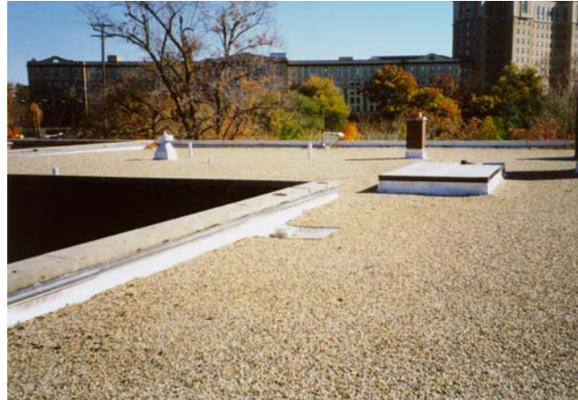
Overview of completed roof replacement.
