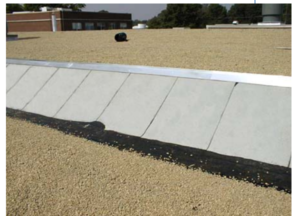
Different slopes and interconnected roof areas were challenges during the project.
