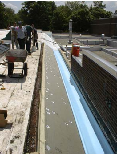
Extensive detailing ensured that all transitions were watertight.
