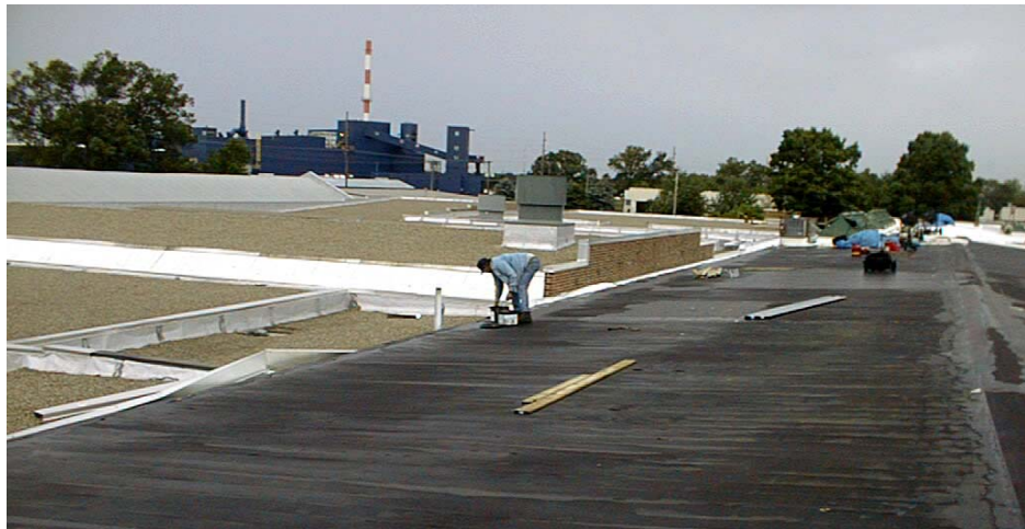
Overview of plant with work in progress.
