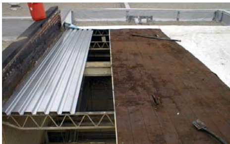
...portions of the deck were replaced.
