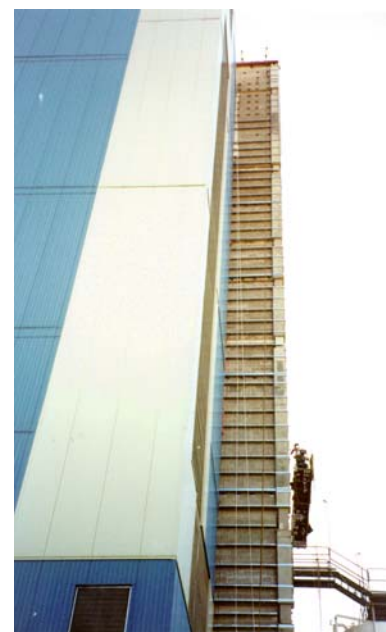
All deficient panels were replaced on the tower.
