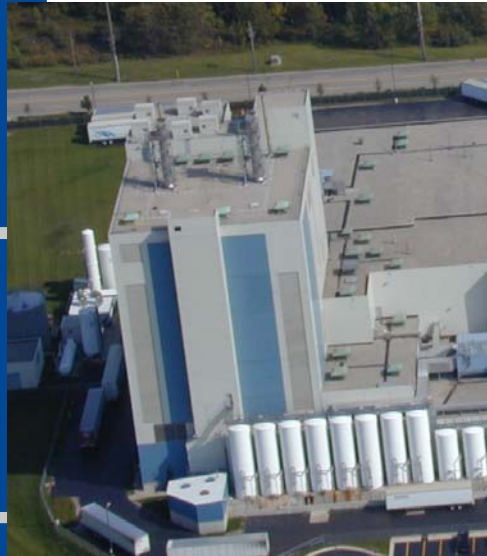
Overview of completed restoration.
