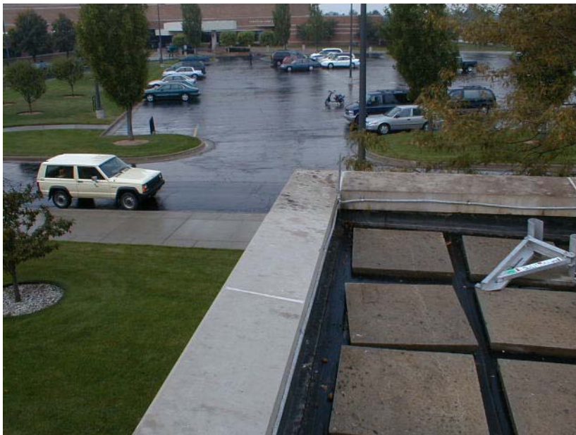
Limestone units being cleaned and prepared for sealant/sealer applications.
