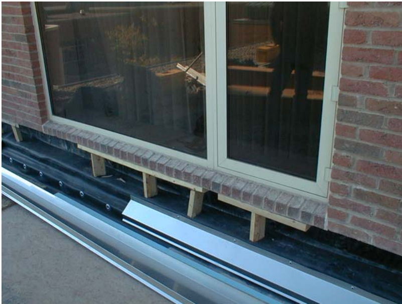
New through-wall flashings installed to correct the water ingress problem.
