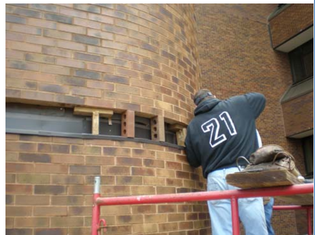
Sheet metal used to conform to the curvature of the masonry
