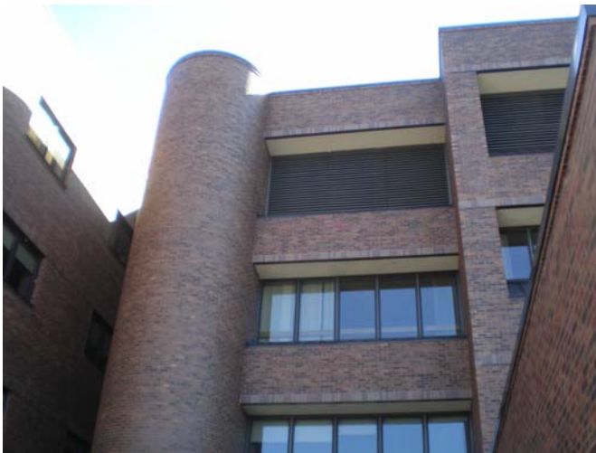
Overview of building envelope post construction
