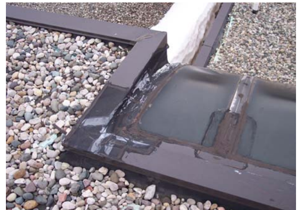
Building transition at skylight termination requiring "attention to detail"
