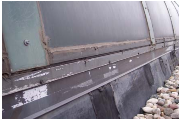
Overview of existing skylight details
