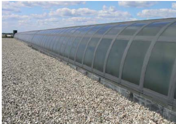
Restored south quarter-barrel skylights
