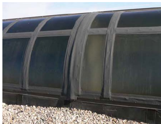
Restored quarter-barrel skylight expansion joint
