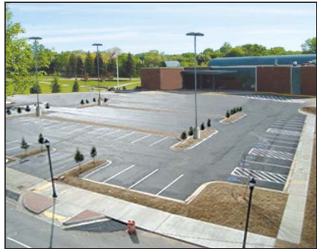
Restored corporate parking lot
