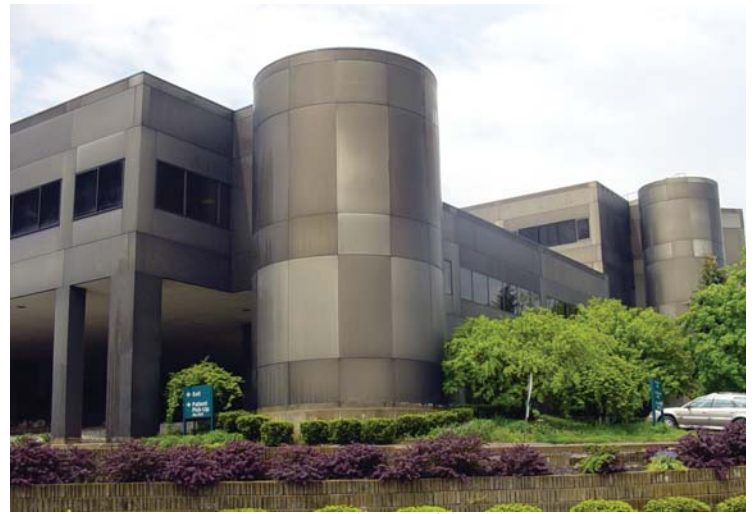
Overview of the 1976 building.
