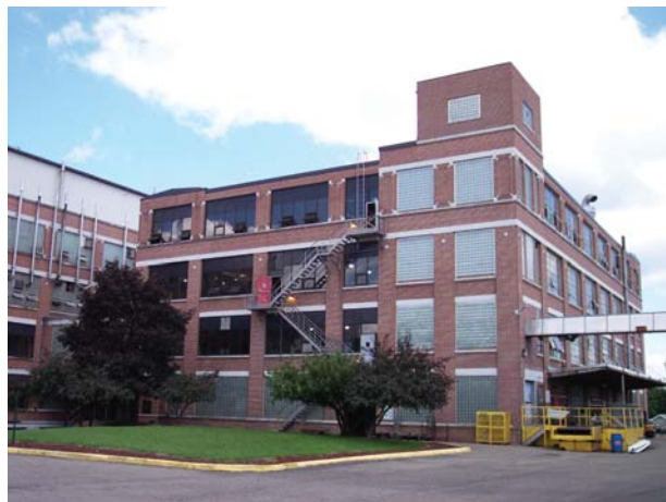
Overview of Kraft - Post Division Complex
