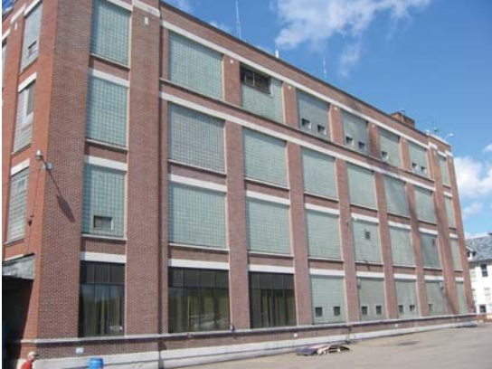
Masonry wall facades dominated the structures of the complex.
