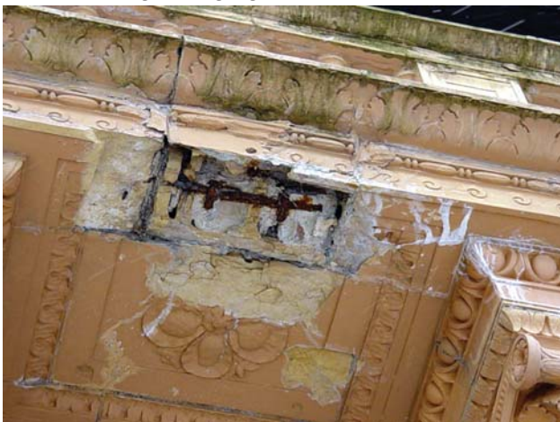
The spalling of the terra cotta on the balcony was caused by the rusting of the embedded steel, as well as extensive freeze/thaw cycles.
