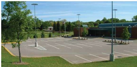
Restored parking lot.
