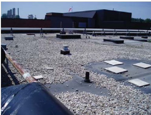
Overview of aged ballasted EPDM single-ply roof system
