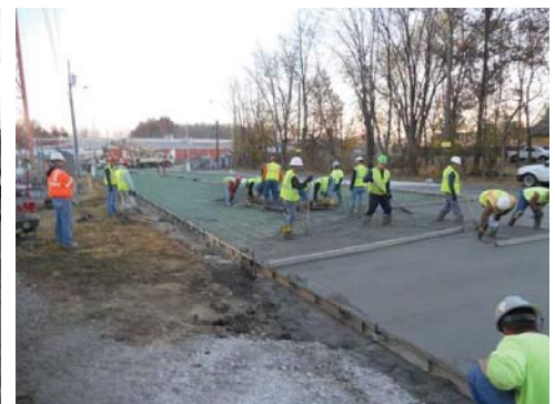
36 ft. wide roadway during concrete pour with finishing crew.
