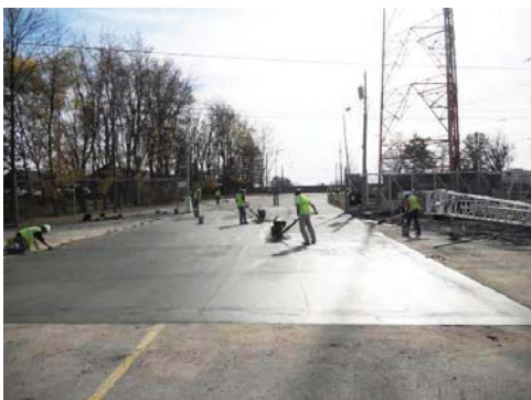
Power trowel finishing for concrete surface.
