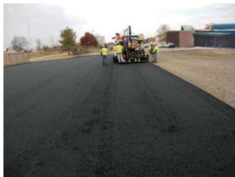
Base course placement pavement section.
