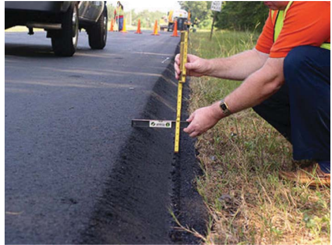
Verification of minimum pavement depth.
