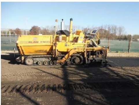
Hot Mix Asphalt laydown paving machine.
