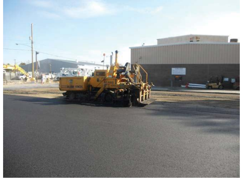
Base course placement pavement section - Hot Mix Asphalt.
