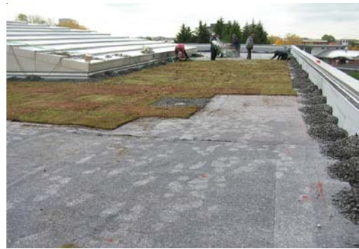
Pre-vegetated mat roof covering being installed
