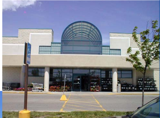
Overview of Davison Store
