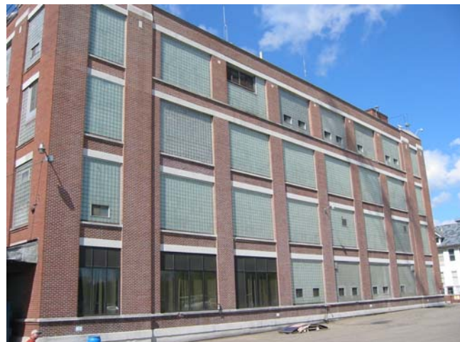
Most of the buildings in this complex have masonry wall facades.
