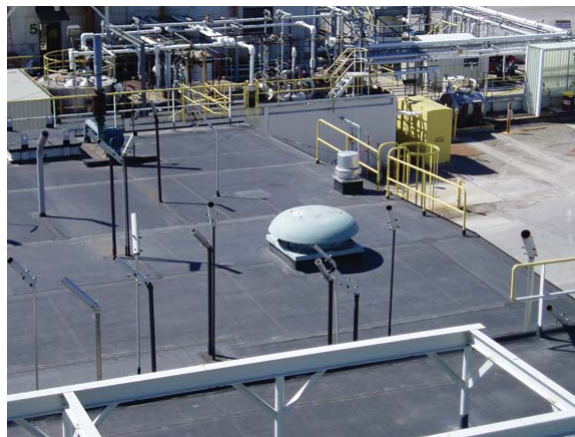
Overview of Roof Top
