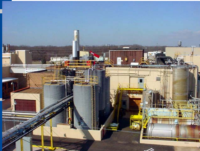
Overview of a portion of the complex.
