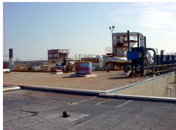
StructureTec had previously helped CDR install new roofs which were inventoried during the evaluation.
