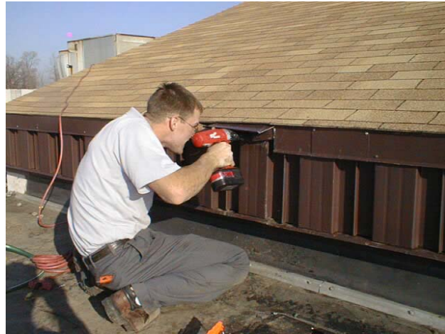
Metal panels were reconstructed to provide watertight integrity.
