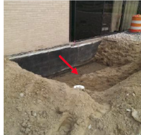
Overview of exploratory excavation at Southeast side of North Tower
