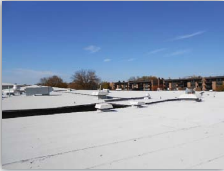
Dirksen Junior High - After Roof Replacement
