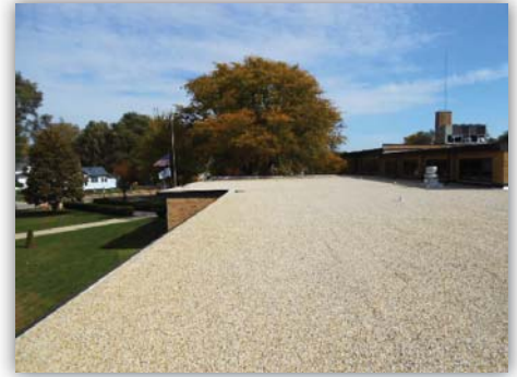
Keith Elementary - After Roof Replacement
