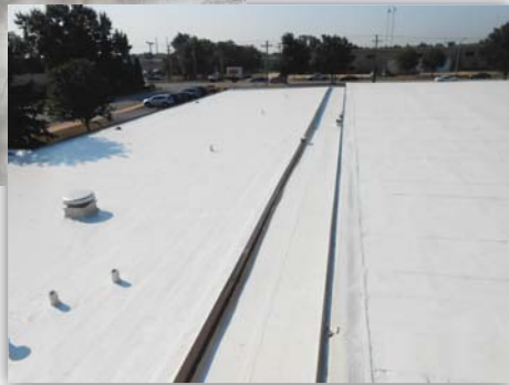
Marycrest Early Childhood Center - After Roof Restoration
