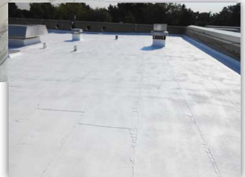
Cunningham Elementary - After Roof Restoration
