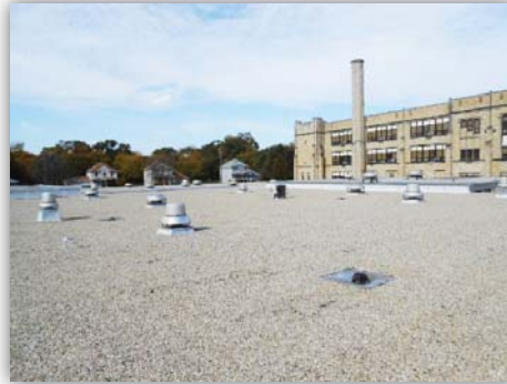
Washington Junior High - After Roof Replacement
