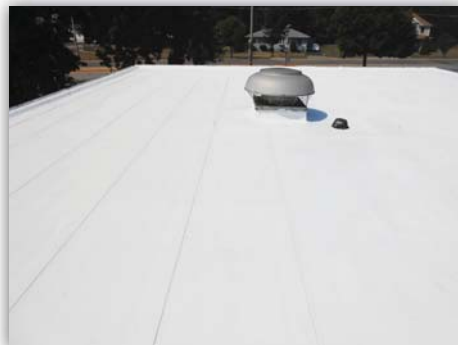
After Roof Restoration
