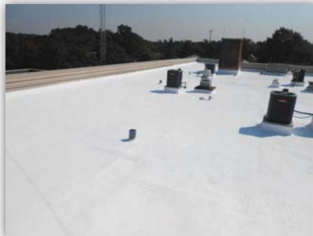
After Roof Restoration
