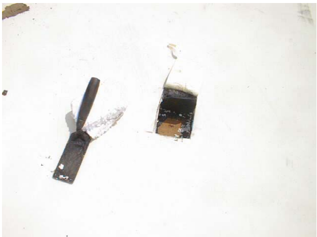
Test cuts revealed overall construction. Retrofitting had occurred and existing insulation appeared saturated.
