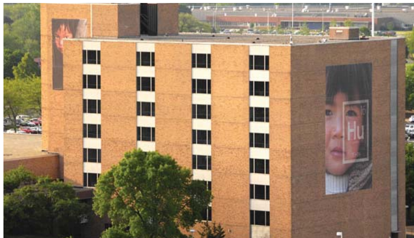
Overview of Dow 2030 Building
