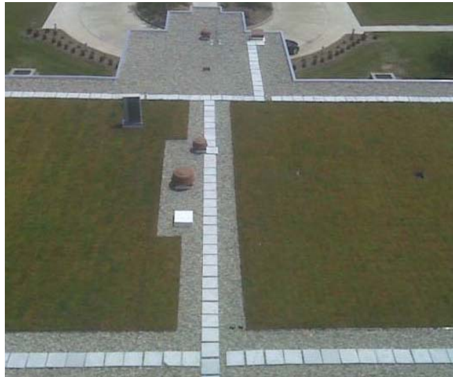
Overview of finished green roof
