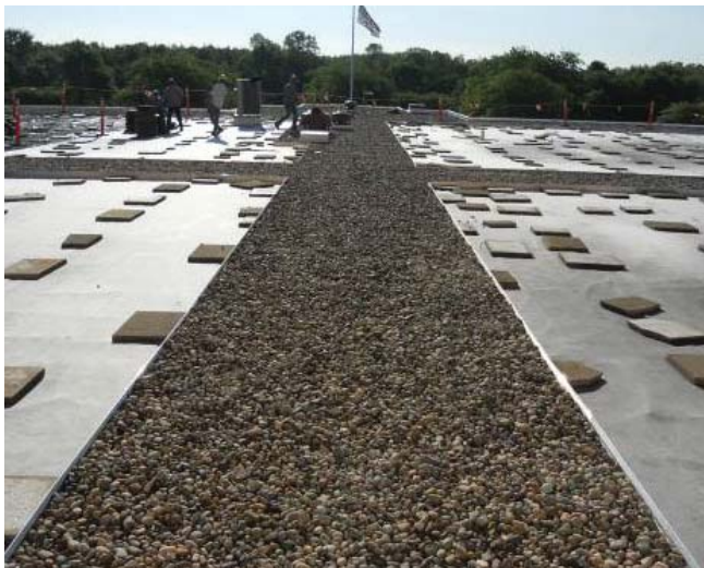
Stone walkway installed before vegetated component
